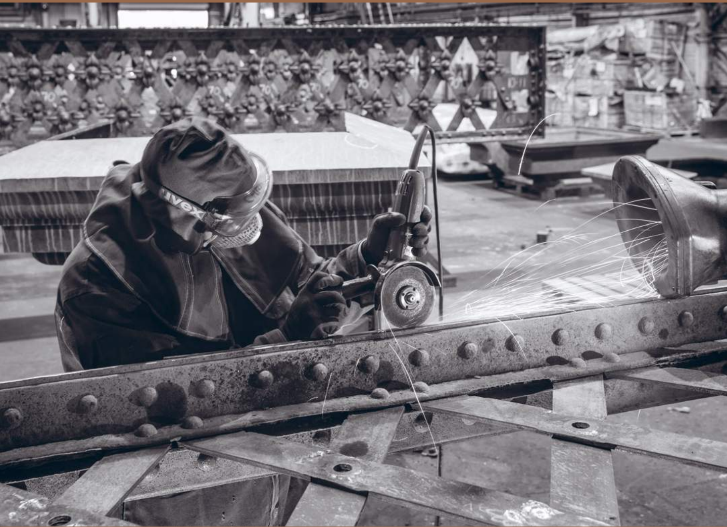
It has taken over two years to painstakingly refurbish the 123 cast-iron gasholders columns
